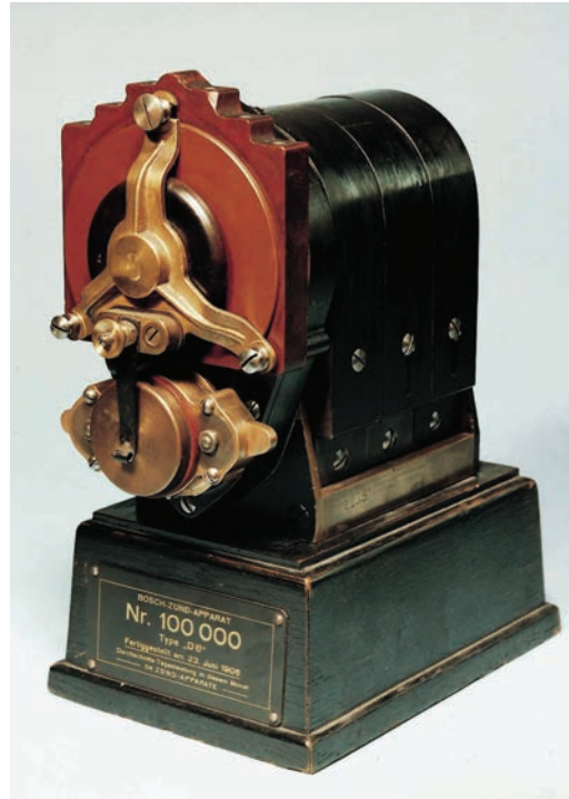
Figure 1.3 Magneto (Source: Bosch Media)
